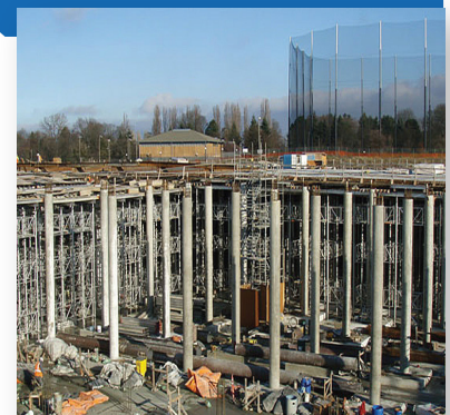
Beacon Hill Reservoir Seattle
