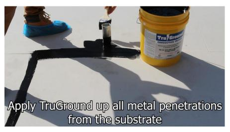
2. If no metallic penetrations are located within the area where **TruGround** is being installed, then a grounding object must be installed. Any metallic object can be fastened to the structural deck and connected to the primer by coating the side of the object with the primer. Flash grounding object with roofing membrane is the same per requirements of the manufacturer.
